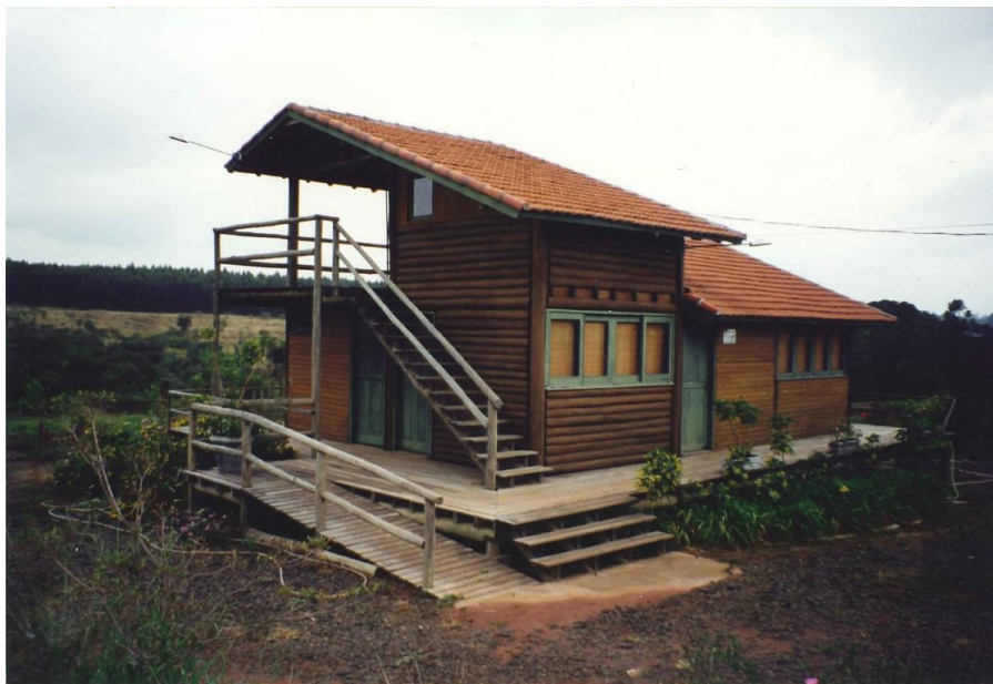
Realization of a project developed by the Habitation Group (Ghab).
